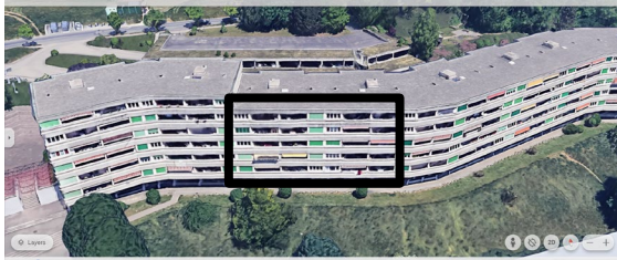
Figure 1: Example building facade with 20 balconies, a summed balcony length of 100 m and a maximum of 40 modules (for max. 2 or 3 modules per apartment). Source: Google Maps.
